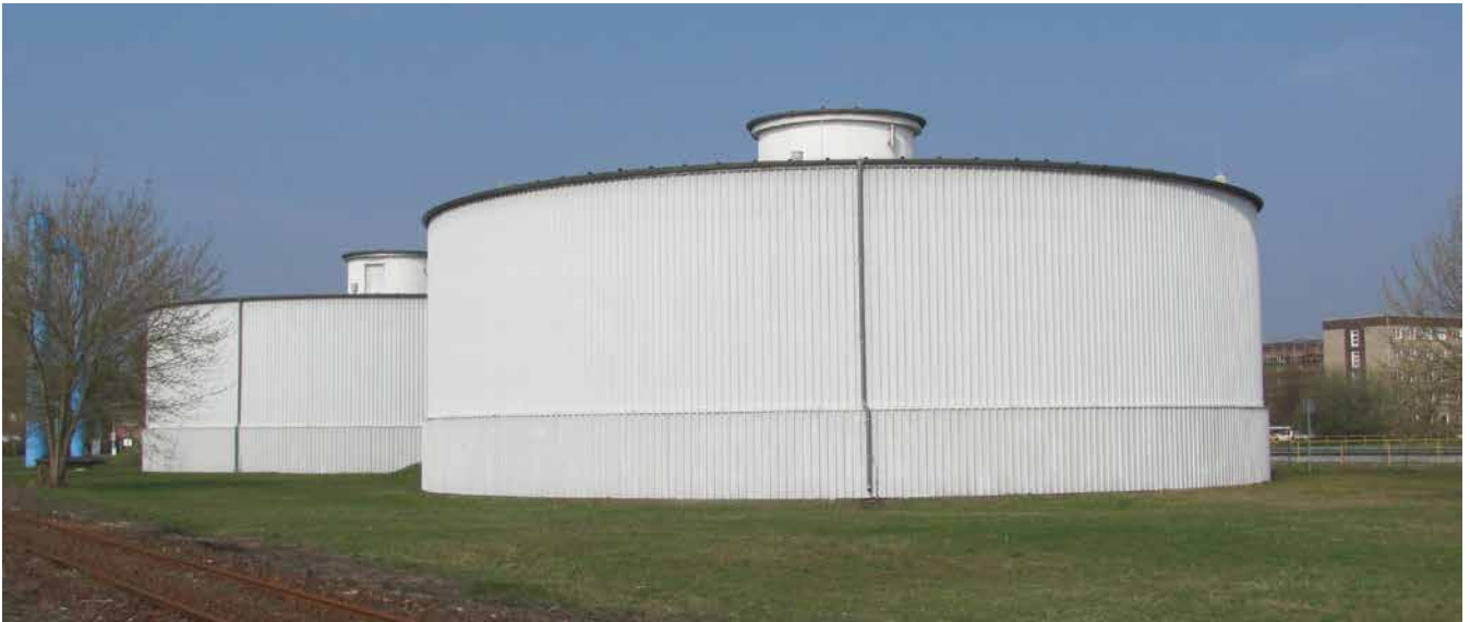
Drinking water tank "Schwarze Pumpe"
