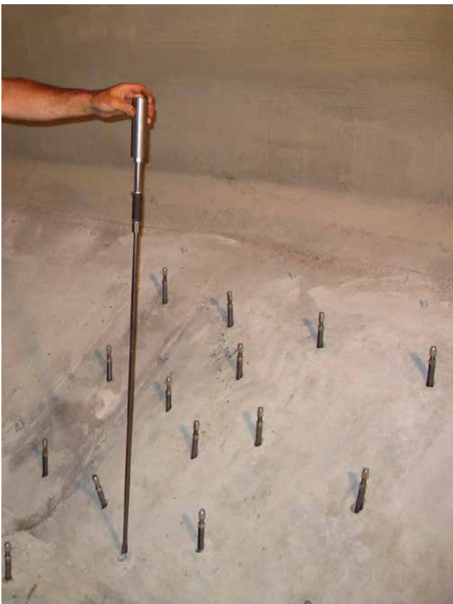
Set ram injection lances – drinking water tank "Schwarze Pumpe"
